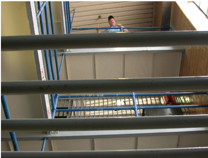
Interior Stairwell Core
