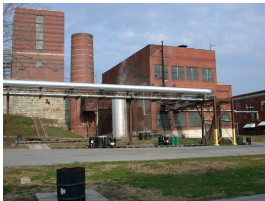
Old Boiler Plant and Overhead Piping
