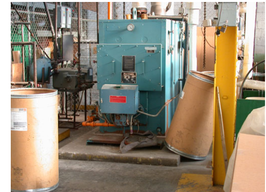
Auxiliary Boiler
