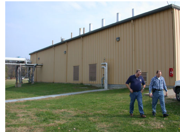
Boiler Plant Exterior
